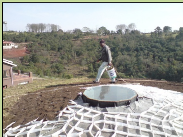
Detail of roof layers and eaves treatment
