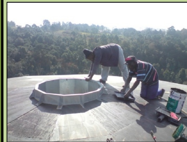
Applying bitumen sealer
